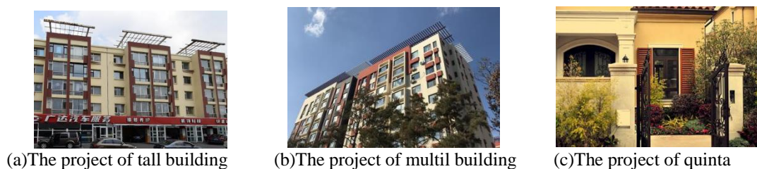
Figure 2: Suspended Plates on the Top of Buildings in Two Communities
