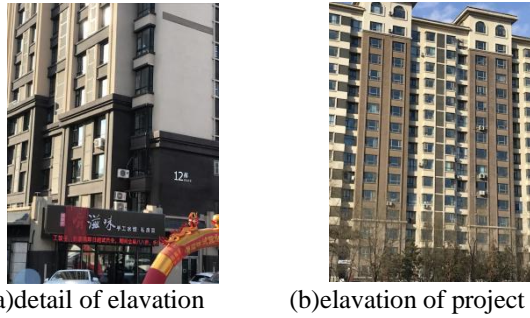
Figure 1: Air Conditioner External Unit Positions in Two Communities
