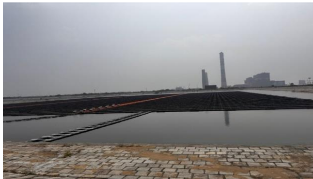
Figure 3: 5 MW Solar Floating PV Plant at SCCL, Jaipur, Telangana.
